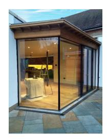
main glass units where supplied in a toughened/laminated specification giving them greater resistance to wind loading removing the need for vertical support and a Burglar resistance rating of P4A to EN356.
